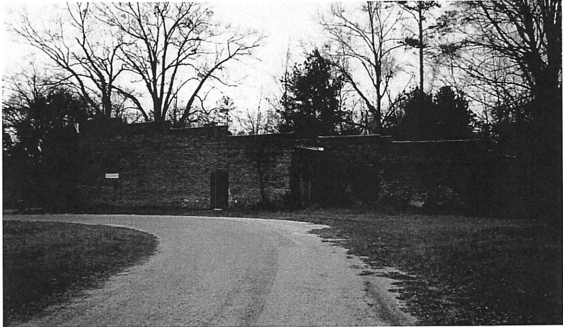
The side of the Durham Mercantile Company. The large door to the far right is the loading dock where farmers would load supplies into their wagons and where Mr. Durham would take in goods brought by train.
